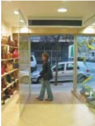
▶ Optima Installation in a window corridor shop
